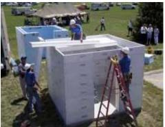
Construction workers build a steelreinforced concrete safe room, which will be placed inside a home. Many safe rooms are prefabricated like this example and are transported to homes throughout the U.S. (cement.org)
