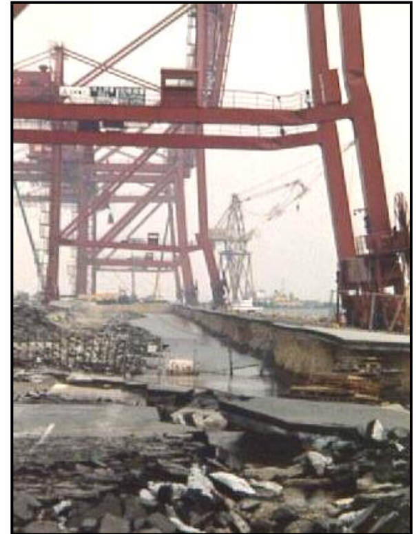
Damage at Port of Kobe: Crane legs buckled, soils failed at container terminal
