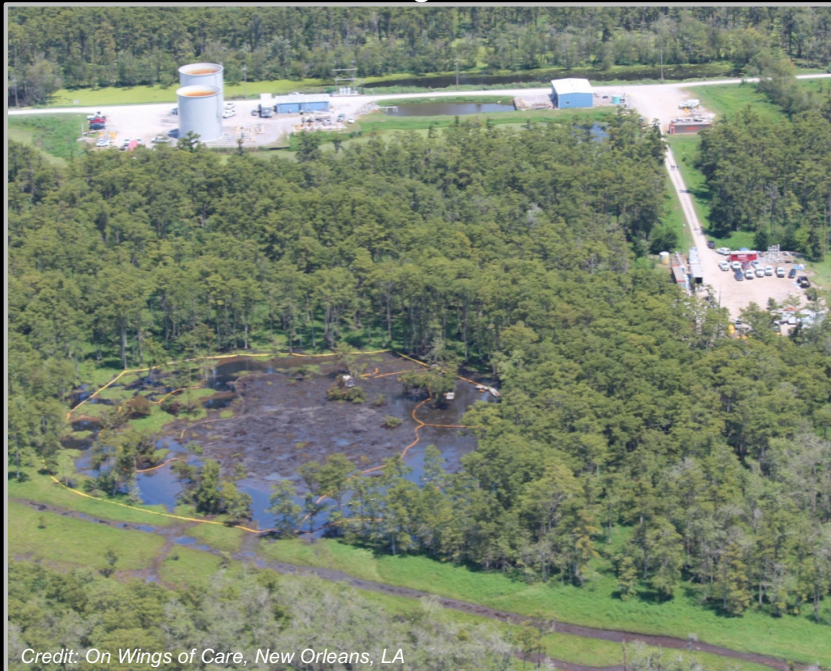
Sinkhole formed on Aug. 3, 2012:
