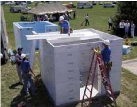
Construction workers build a steel-reinforced concrete safe room, which will be placed inside a home. Many safe rooms are prefabricated like this example and are transported to homes throughout the U.S. ([cement.org](http://www.cement.org))
